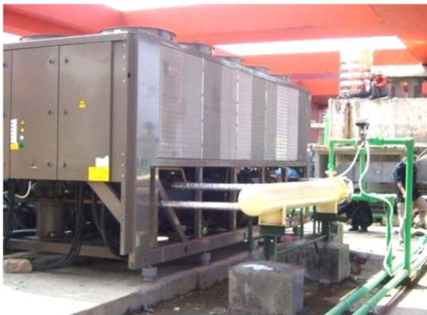
Heat recovery from refrigerant hot gas to water .
